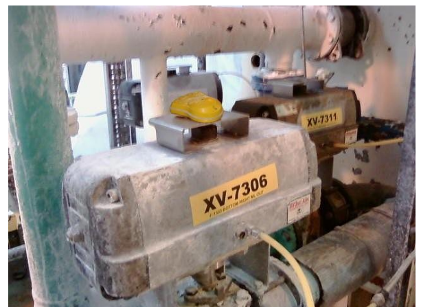
Eltav’s VD Installed on an Actuator
